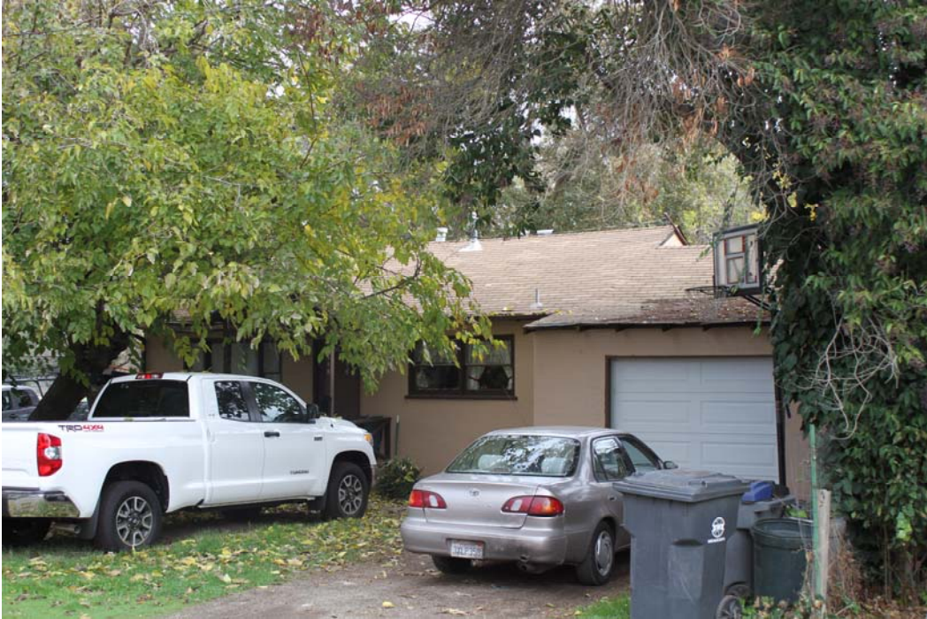
Figure 23: 118 Hickory Lane residence, looking notheast from Hickory Lane.
