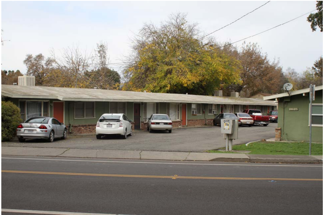
Figure 14: Kober Apartments, formerly the Kober Motel, 1225 Olive Drive, looking north.
